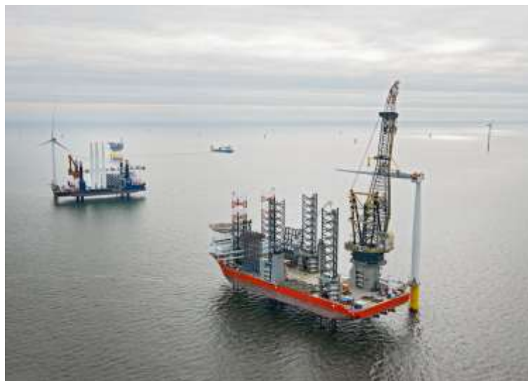
Figure 5-3 Installation vessel used in Gemini wind farms (Source: https://geminiwindpark.nl/turbines--nacelles--rotorblades.html )
